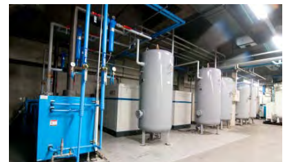
Variable-frequency and full-frequency air compressors
