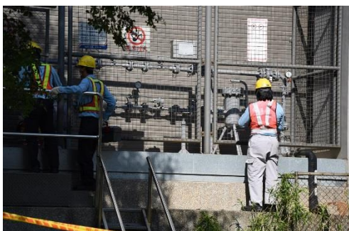
Repairing natural gas leak
